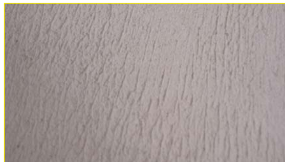
Wood Float Finish
